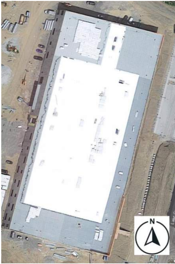
Figure 1: 33 Jackson Rd. Aerial View
